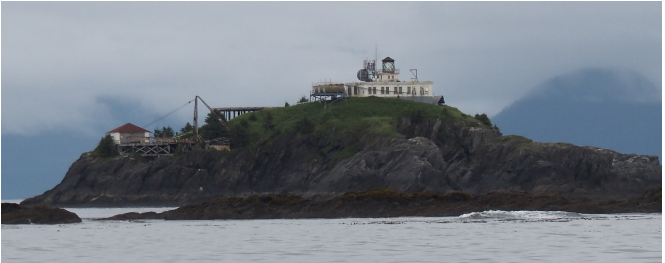
Cape Spencer lighthouse greeted us as we made landfall from the Gulf of Alaska
