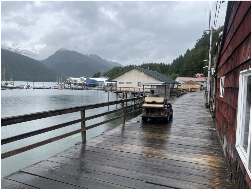
Almost the whole of Pelican is built on pilings
