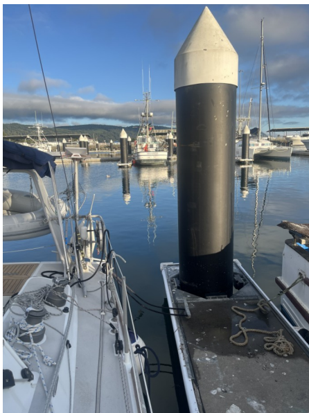
Piles designed to survive the next tsunami
